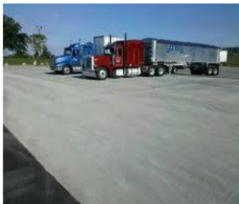
Trucks parking yards made of RCC
