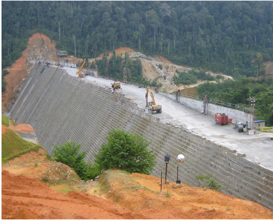
Fig. 14- Construction of RCC Dam in end levels of construction
