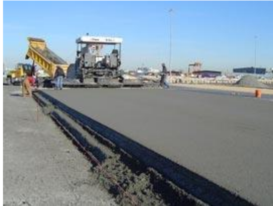
Using Ordinary Trucks and Paver
