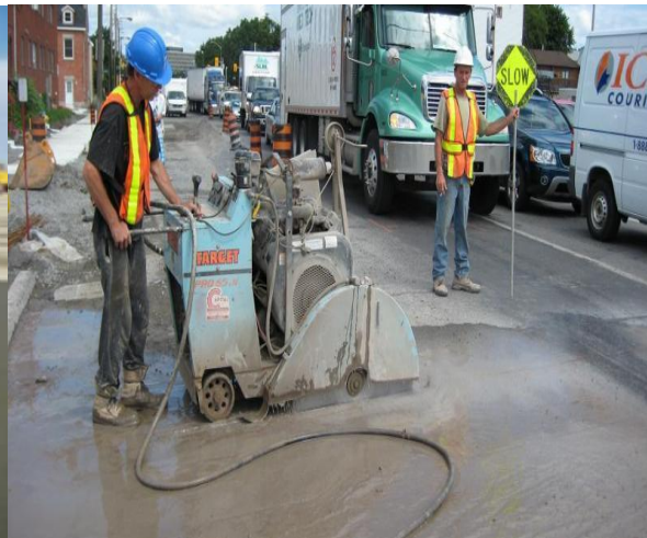
Fig. 16- Constructing the joints after layering
