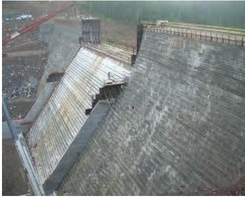
Construction of RCC Dams
