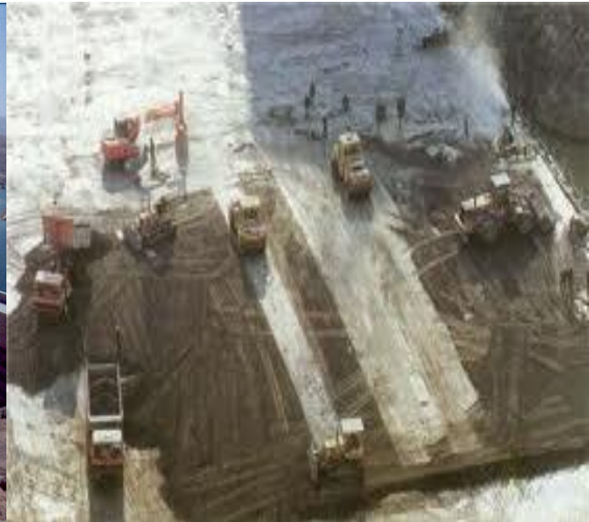
Fig. 10- Construction of RCC dam in initial progress of works
