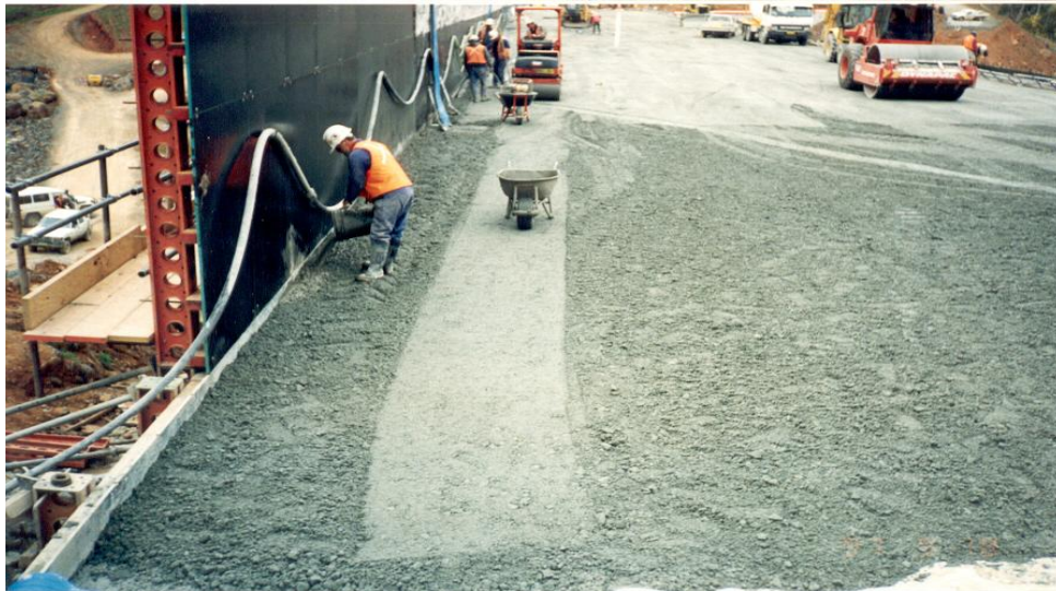
Fig. 13- Adding additives to the surface of the concrete forms in dam in order to smooth surfaces
