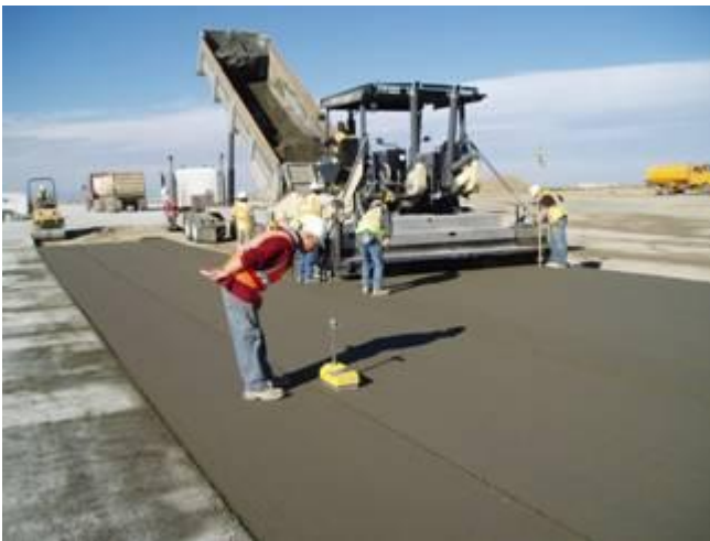
Fig. 15- Testing the density of compacted concrete of the road
