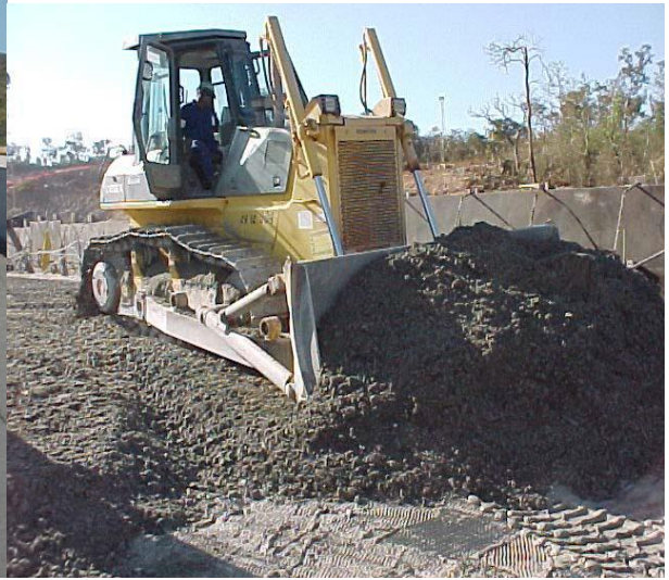
Fig. 8- Using Bulldozers to layering the concrete
