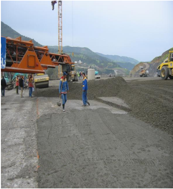
Fig. 11- Layering suitable grout between the pavement layers
