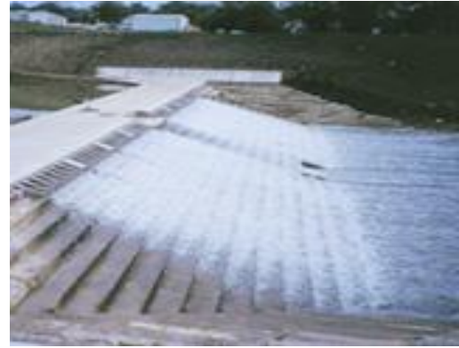
Construction another type of RCC Dams
