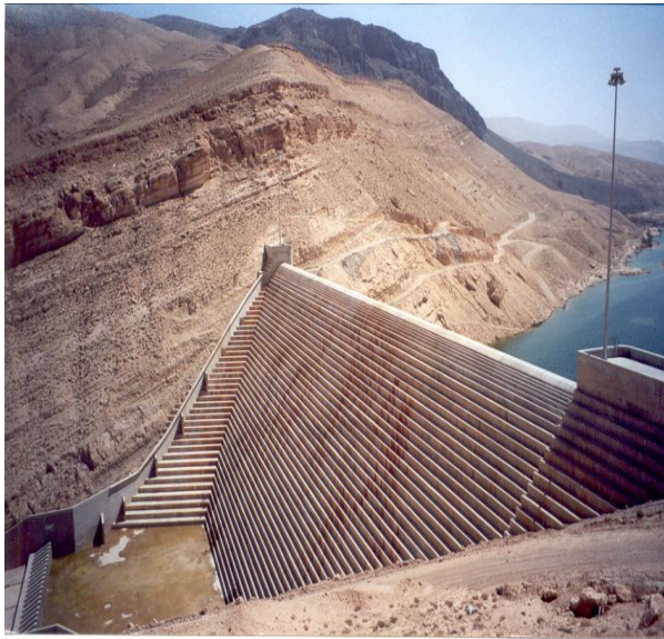
Fig. 9- Constructing RCC Dams by using layer by layer concrete paving
