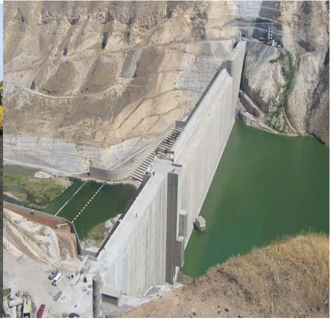
Fig. 12- RCC Dam after completion
