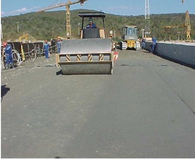
Fig. 7- Vibratory compactor Used for RCC Paving
