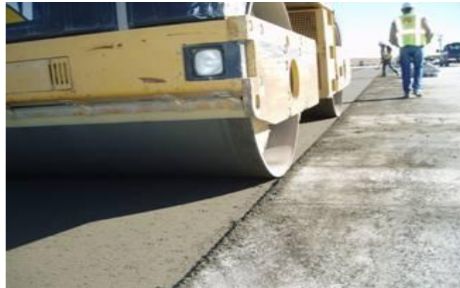
Using ordinary Roller compacter
